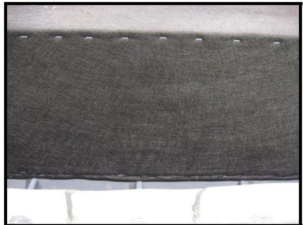
Nonwoven Fabric Silt Fence
