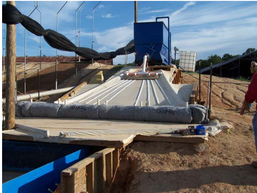
Figure 1. SRD Installed Along and Above Wooden Box Trench
