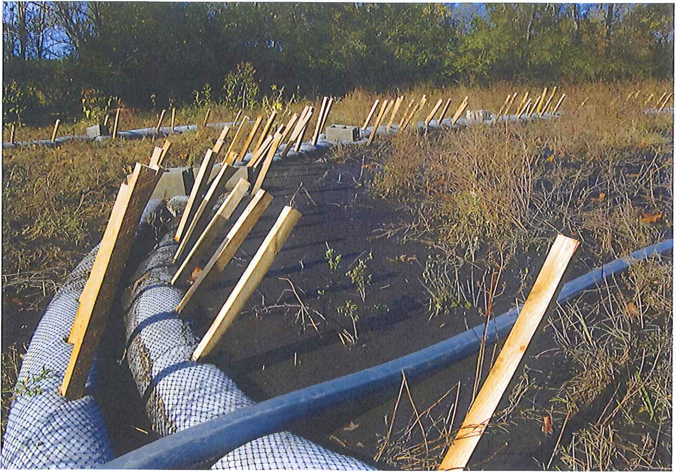
REPURPOSED WASTE MATERIALS ARE USED TO TRAP SILT PUMPED FROM THE SPRING BOTTOM.
